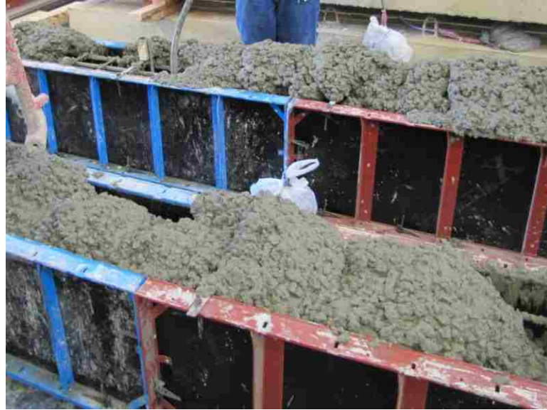
Figure 4.12 Casting of Beam Splice Specimens
