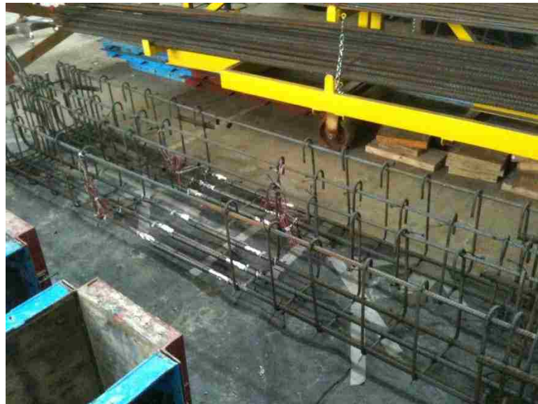
Figure 4.10 Completed Cage for Beam Splice Specimen
