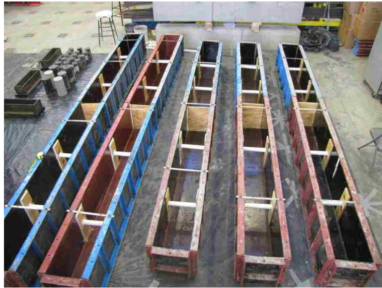
Figure 4.1 Formwork for Casting Pre-Recycled Concrete
