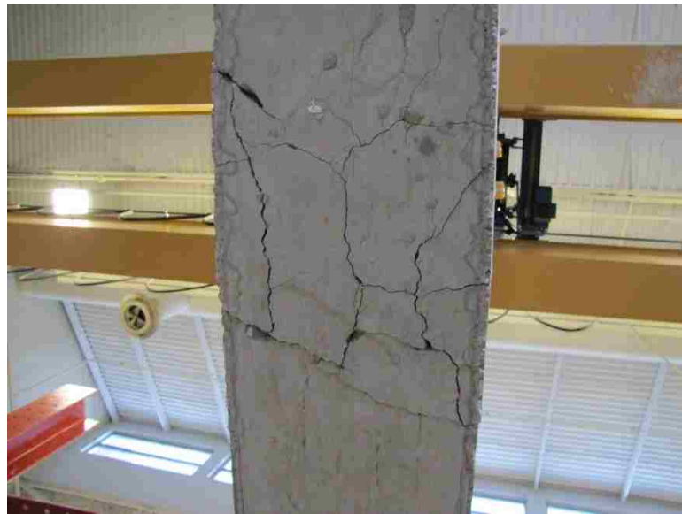
Figure 5.14 Beam Splice Specimen Bottom View at Failure (RAC50-1)
